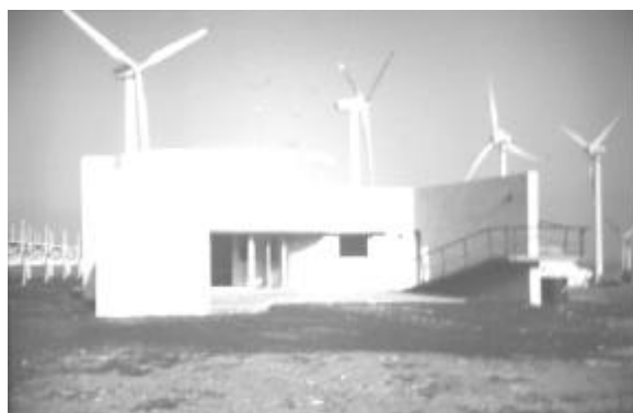
Fig. 9: Control building and visitors centre with the meteorological station at the top.
