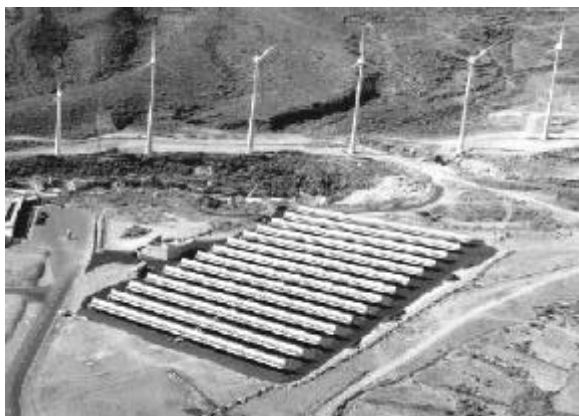
Figure 1: Aerial view of the EUCLIDES Plant installed in the grounds of ITER in Tenerife (Canary Islands, Spain)
