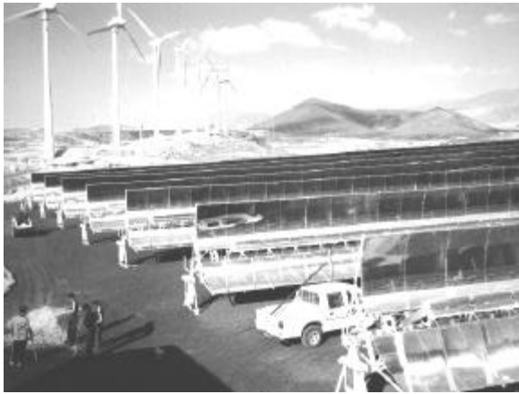
Figure 3. A partial view of the PV field during initial operation set-up.
