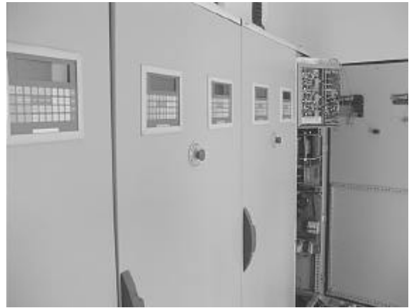
Figure 4: The seven TEIDE inverters for the fourteen arrays.
